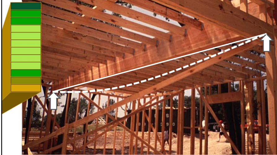
Simple Span – Unbalanced Layup
