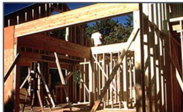
Simple span beam
