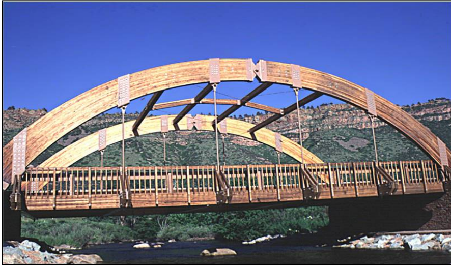
Glulam Arch Highway Bridge Suspended Deck - Colorado
