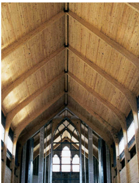
Church, Palm Beach Gardens, Fla., Unit Structures
